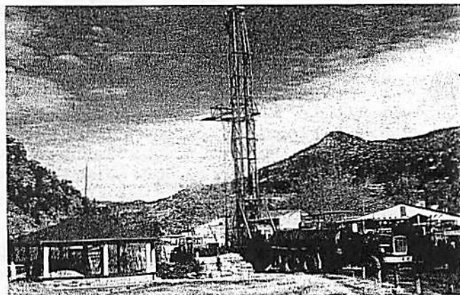
FIGURE 1.33. Drilling an exploratory geothermal well (1978–1979) in Jemez Springs town, mile 71.4.
